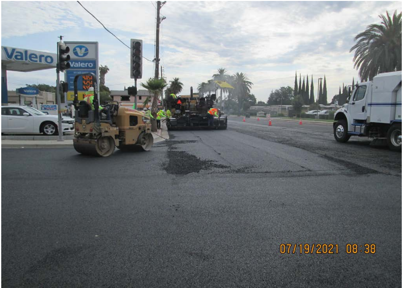
Paving at Las Palmas Avenue and First Street
